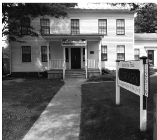
Berkshire Free Library awaits its new roof
