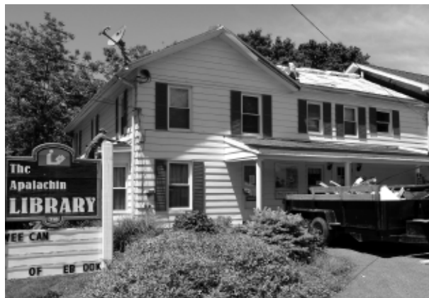
New roof in progress at the Apalachin Library
